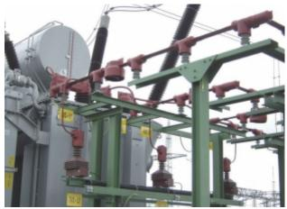
Substation equipment is vulnerable to flashovers caused by accidental bridging of phases, or phase to earth. Usually made by birds, animals, vegetation or airborne debris, flashovers can be very expensive in terms of damage to equipment, reduced reliability and in some cases even electrocution of protected species. Almost any event of this nature can be prevented by insulating the strategically vulnerable bare metalwork with a combination of Raychem Raysulate products.
