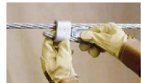
Place tap on conductor
