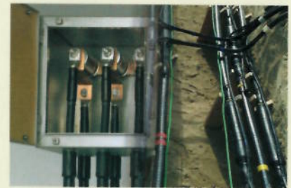
Cross-bonding Design and Installations
