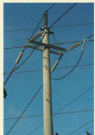
Installation of Covered Conductors
